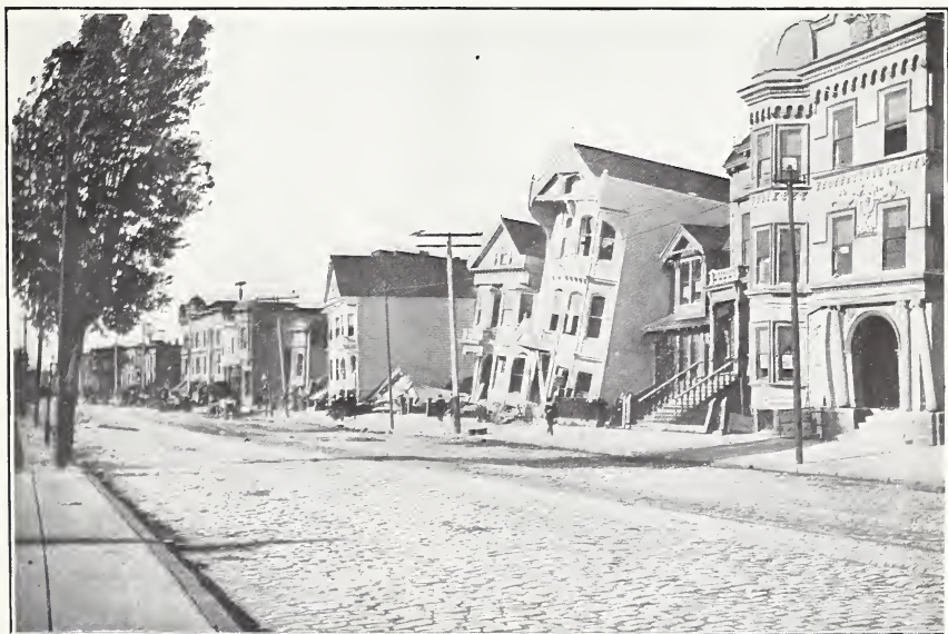
B. GENERAL EARTHQUAKE EFFECT ON FRAME BUILDINGS SITUATED ON ALLUVIAL SOIL, HOWARD STREET, SAN FRANCISCO.
